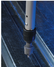
2. Drill Deck Holes
